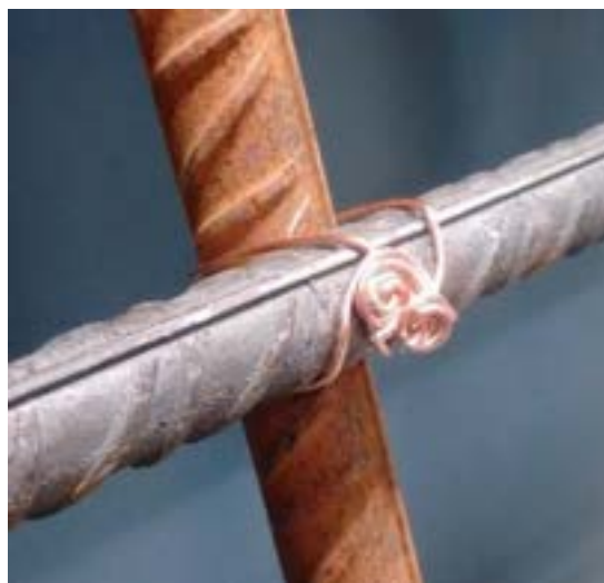
Figure 59 - Close-up on a knot tied by a Knut 39
