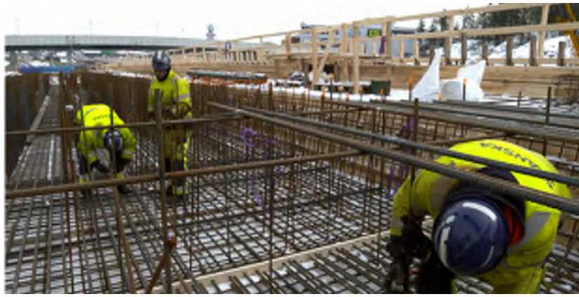
Fig. 1. Manual reinforcement installation in progress.
