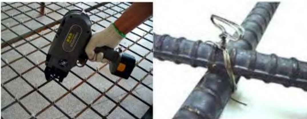
Figure 3 Example of a power-driven tie wire gun and an example of the result when the tie wire gun is used (Kettil, 2012)
